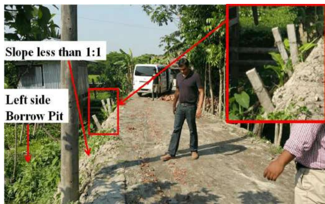
Figure 8 Steep side slope of rural roads in the study area (Location: Uttarpara, Uzirpar, Barishal).
