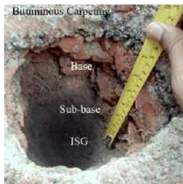
Figure 31 Verification of pavement layer thicknesses by making hole on road pavement.
