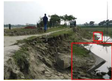
Figure 26 Palisading failed.
