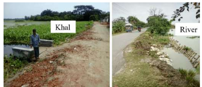
Figure 10 Road along (a) khal and (b) river.
